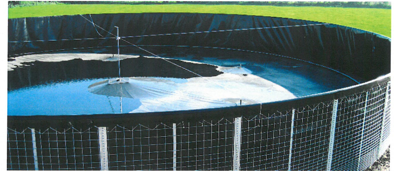
Floating Roof System
